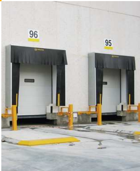
Fixed Dock Shelters installed directly onto the façade.
