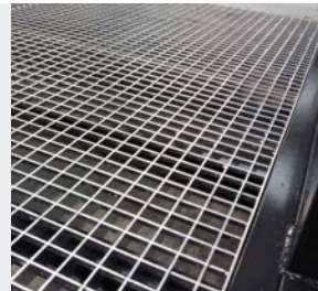
Tramex surface of the ramp.
