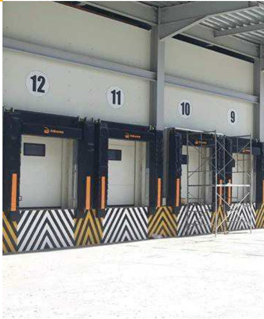
The range of movement of the ABFM's upper canvas is 1000mm.
