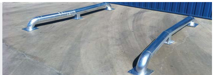
Wheel guides make it easier for vehicles to enter the loading docks, and they protect them from possible knocks.
